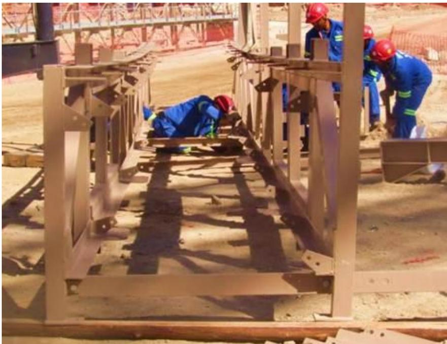
Figure 3. Gantry being pre-assembled
