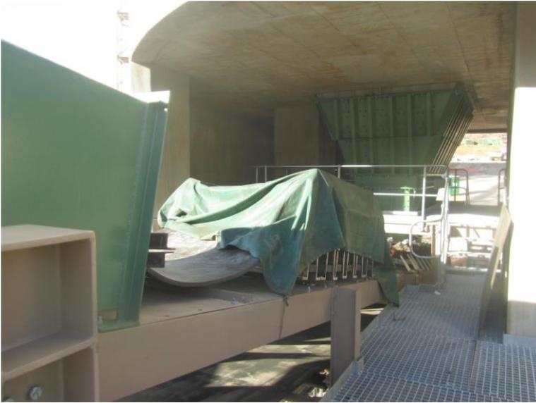
Figure 8. Splicing - hot vulcanisation in progress
