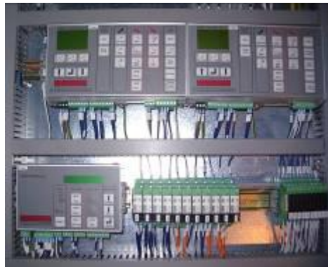
Illustration 28 - two SOBO V4 controllers for Shadow Braking
