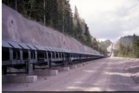
Illustration 20 - overland belt conveyor at the Henderson Mine
