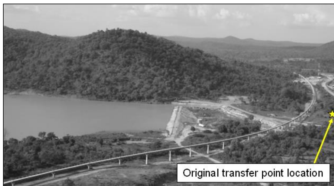
Figure 4 – 2,000m horizontal curve eliminated a transfer point by combining two conveyors
