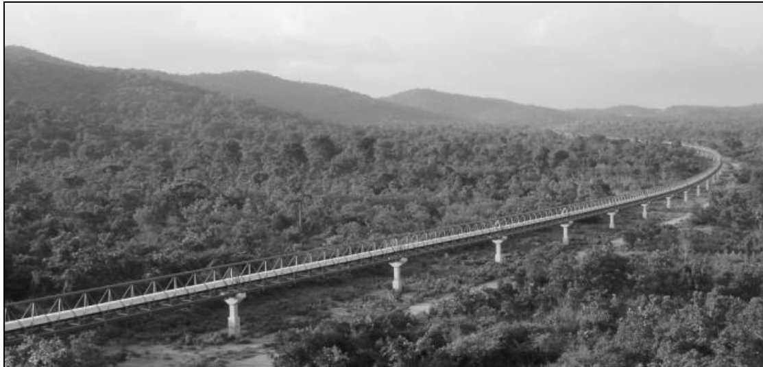
Figure 2 – 6.9km overland conveyor, which is entirely elevated using a triangulated gantry
