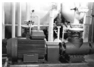
Fig 2: A typical high speed pump drive
