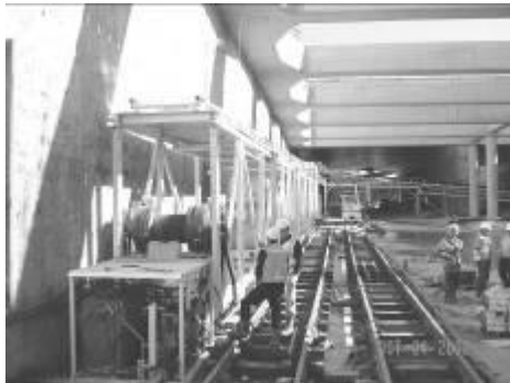
Fig 14: Belt tension unit on CTRL 6.5 Km tunnel with 660 m 12 lap loop storage unit
