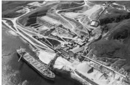
Fig 24: Foster Yeoman - Glensanda operation has used Direct hydraulic drives on its 1850 meter long main conveyor
