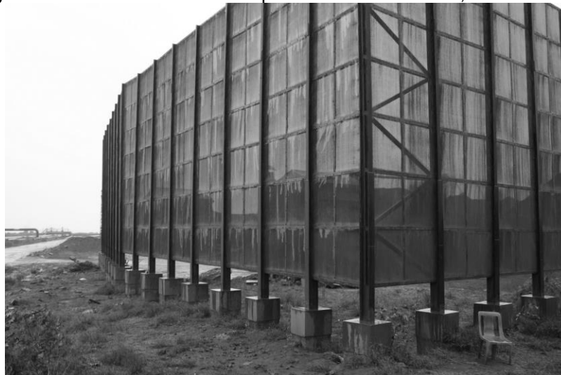
Figure 16: Wind screens in use on the iron ore exporting terminal in Chennai, India.
