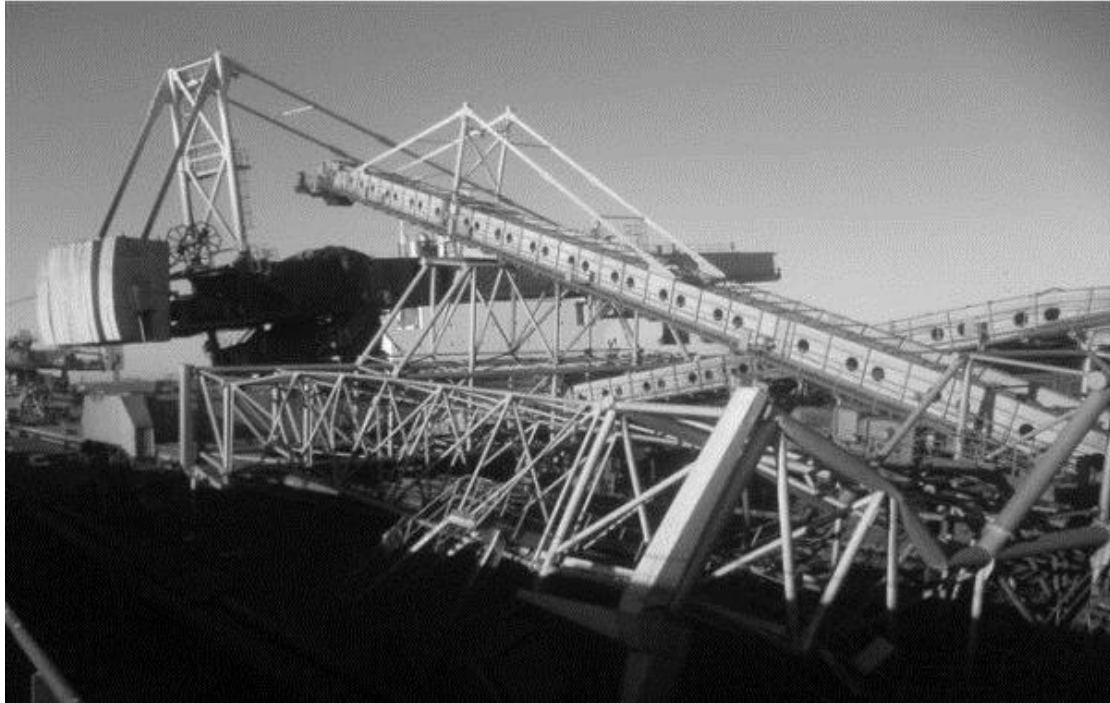
Figure 4.5 – Machine Failure May Have Been Caused By a Blocked Chute
