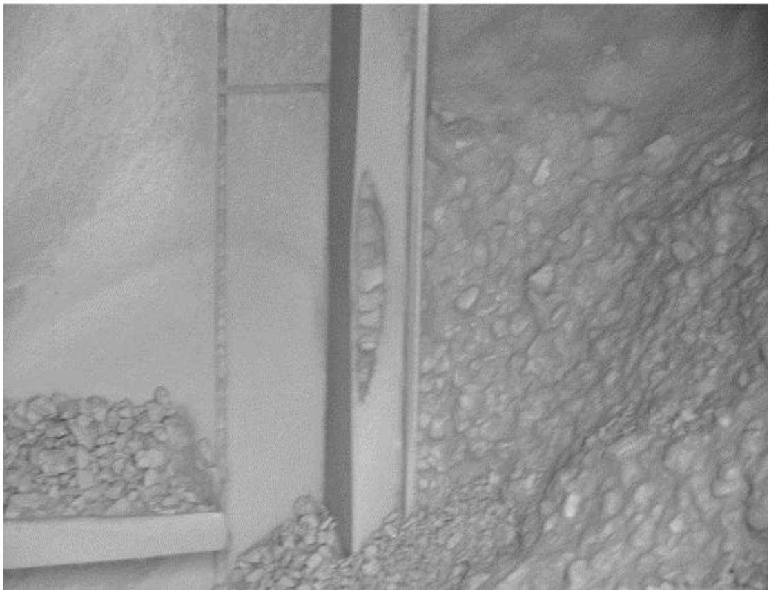
Figure 5.2 – Vertical and Horizontal Shelf Liner (Note the Abrasive Wear Areas)
