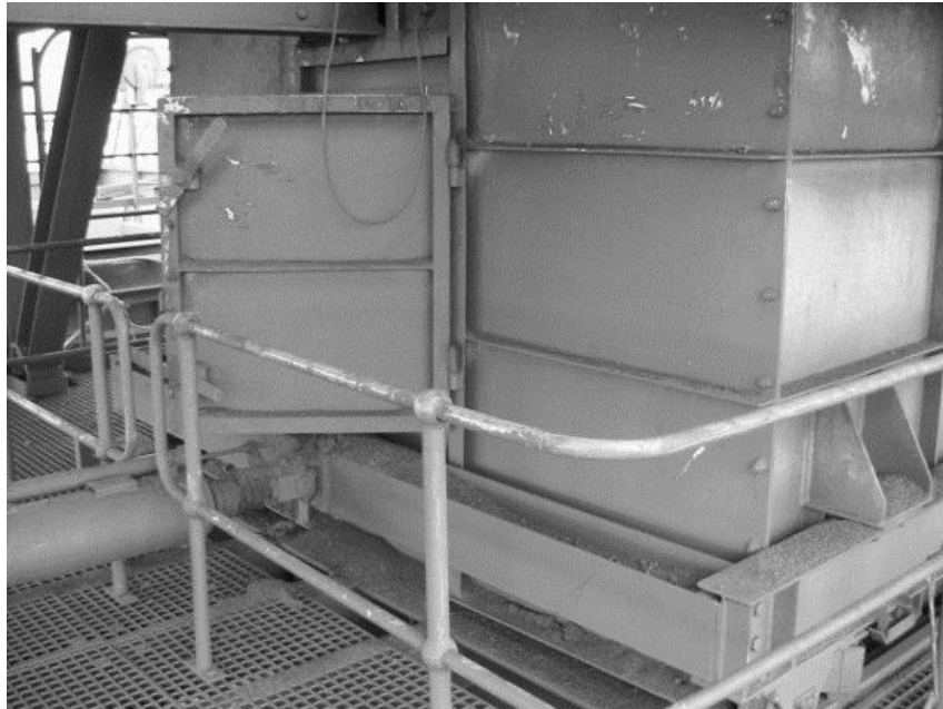
Figure 6.2 – Man access doors for maintenance
