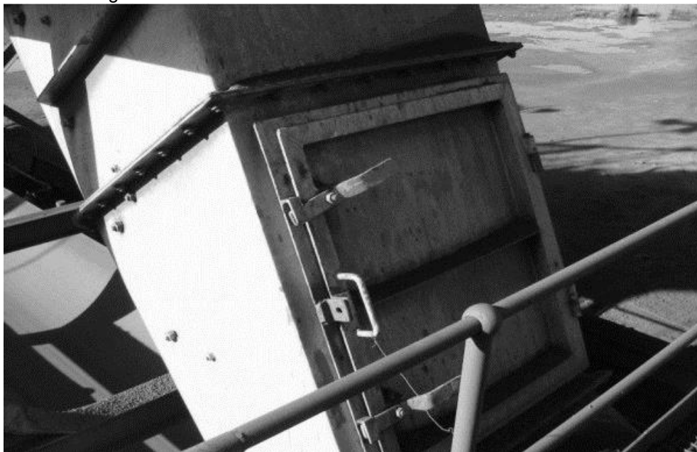
Figure 6.1 – Man access doors for maintenance
