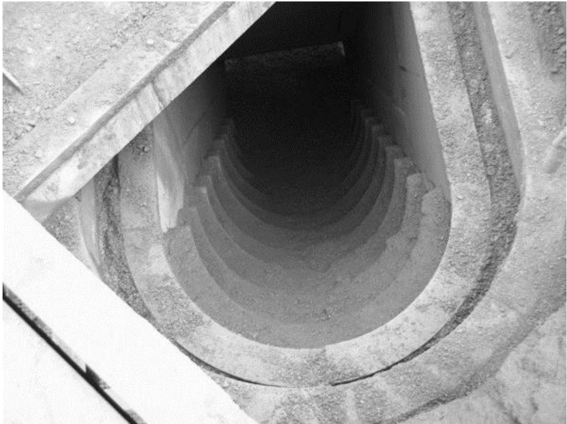
Figure 5.3 – Funnel Design Step Chute (Used to centre material in long drop areas)
