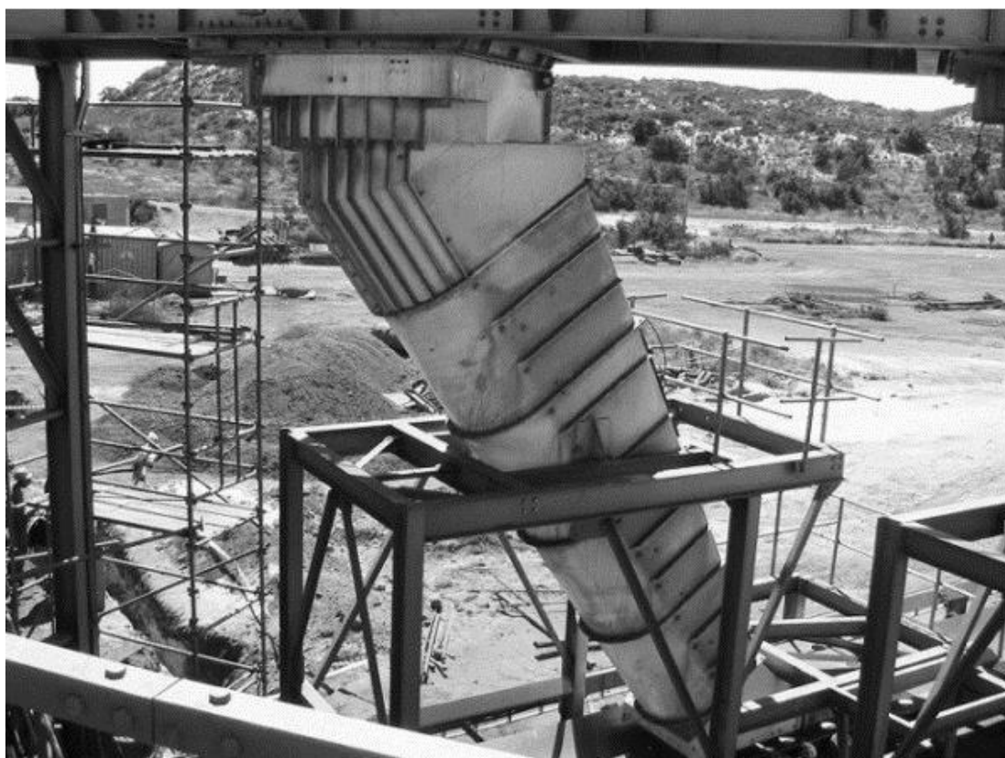
Figure 7.1 – High chute design to accommodate layout constraints
