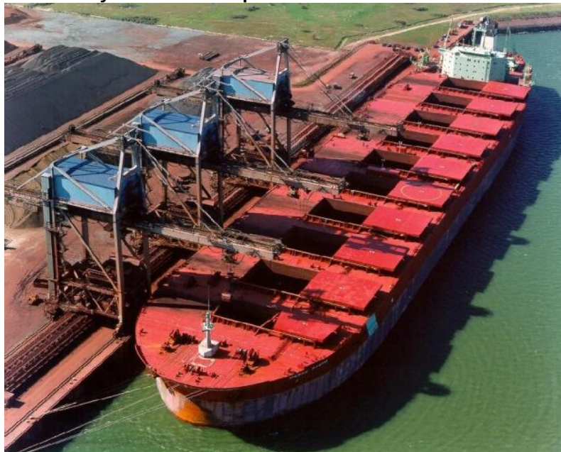
Figure 15: Three ship unloaders working simultaneously on one CapeSize vessel
