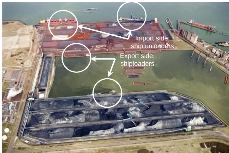
Figure 14: Marine system on the import side and a marine system on the export side of a bulk terminal
