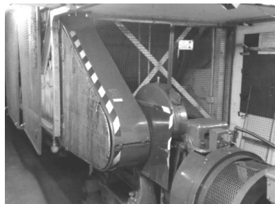
Figure 15.1: Chain driven escalator monitored by MCM
