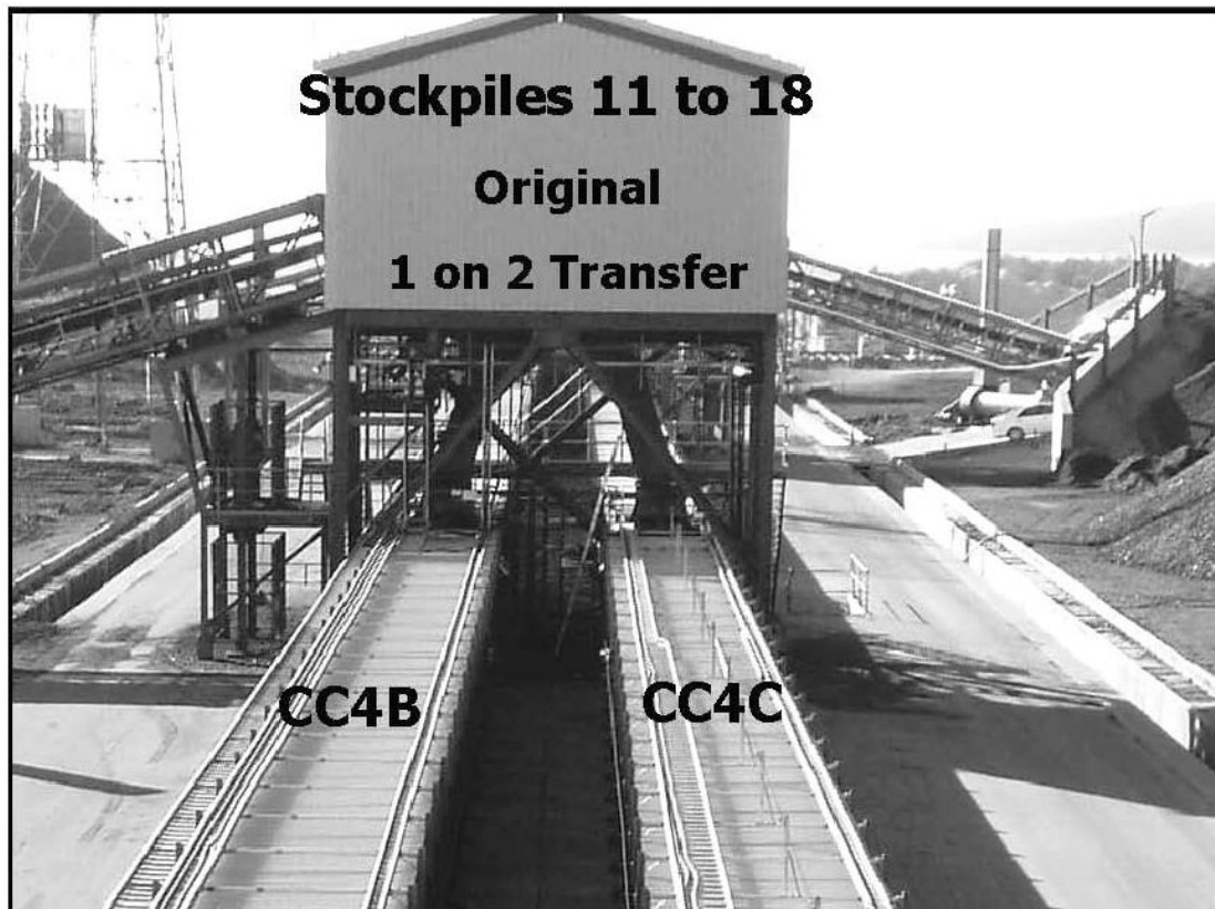
Figure 11. Typical reclaim conveyor to Shipping streams 1 and 2 yard conveyors (typical of Stockpiles 11 to 18/Stockpiles 1 to 10 similar)
