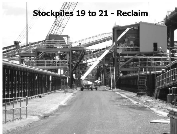
Figure 20. View of Stockpiles 19 to 21 reclaim towers from service road
