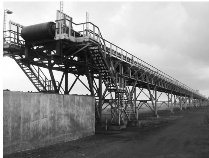
Figure 6. CV731 Wharf conveyor extension
