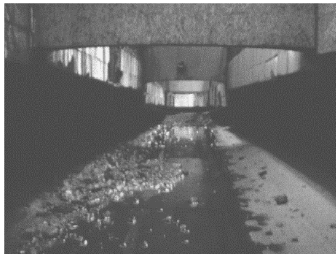
Figure 19. CV404 hopper inside
