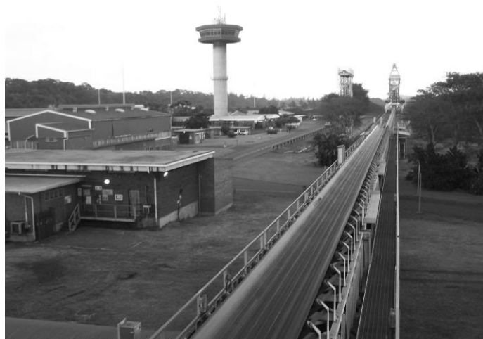
Figure 2. CV610 New stockyard conveyor
