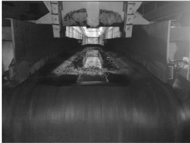
Figure 20. CV013 hopper inside
