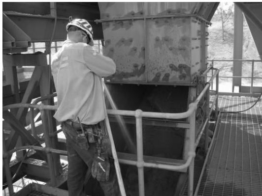
c) Constant house-keeping to remove compacted bed or unblock the chute
