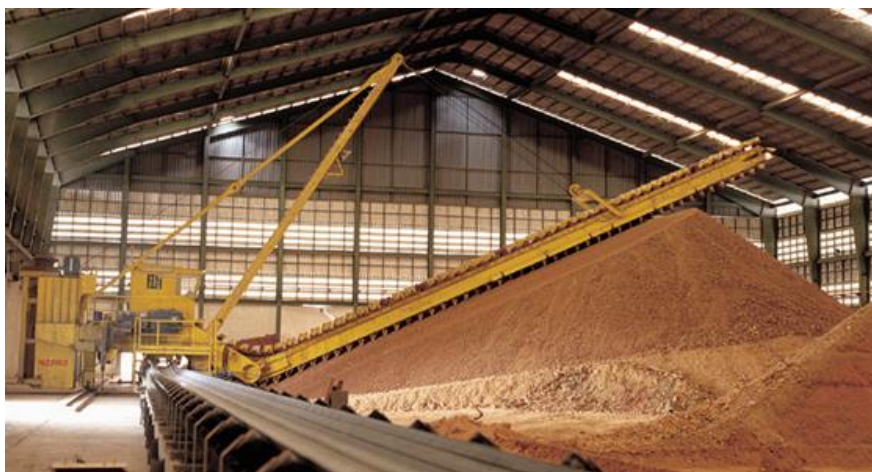
Figure 4. Side arm scraper chain reclaimer
