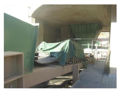
Figure 8. Splicing - hot vulcanisation in progress
