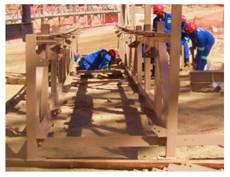
Figure 3. Gantry being pre-assembled
