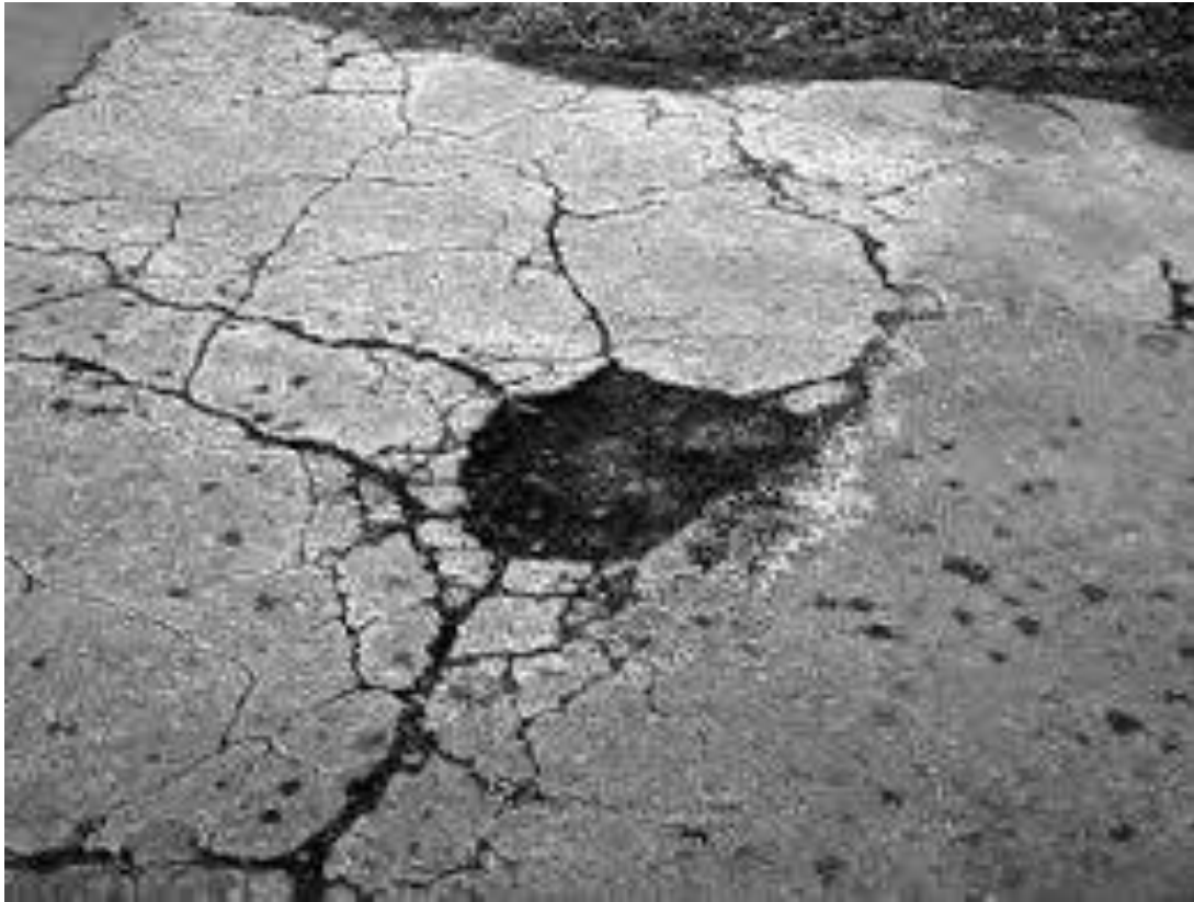
Figure 2. Typical pothole
