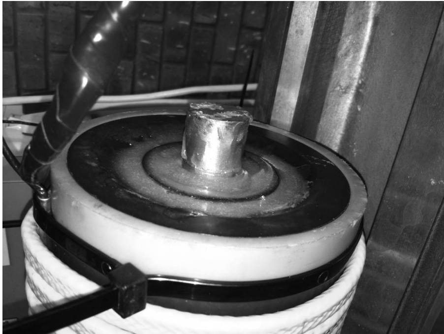
Figure 8. Epoxy sealed bearing
