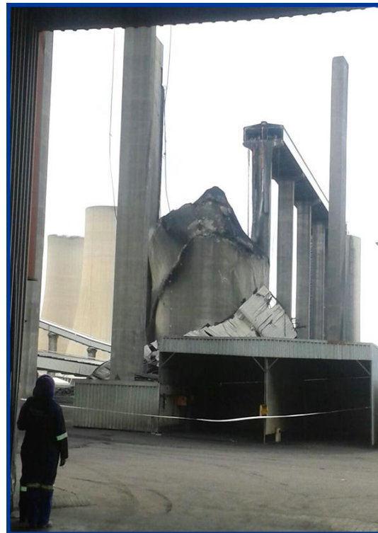
Figure 3. The collapsed silo with the bottom part below the 28 m level remaining in situ.
