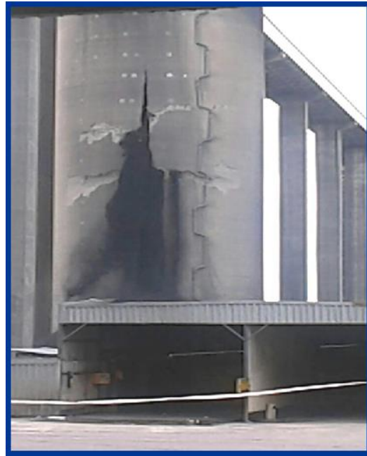
Figure 2. The vertical crack in the silo with coal running from the crack, followed by the horizontal cracks.
