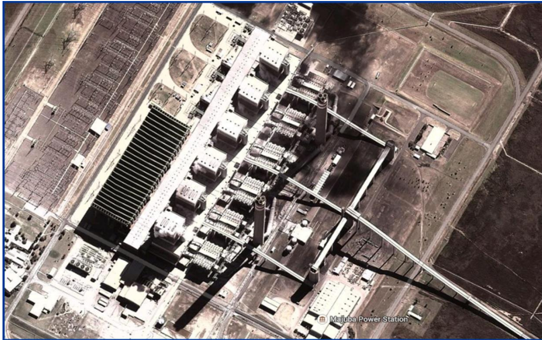
Figure 1. Aerial photograph of the Majuba Power Station.
