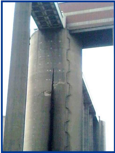
Figure 2. The vertical crack in the silo with coal running from the crack, followed by the horizontal cracks.
