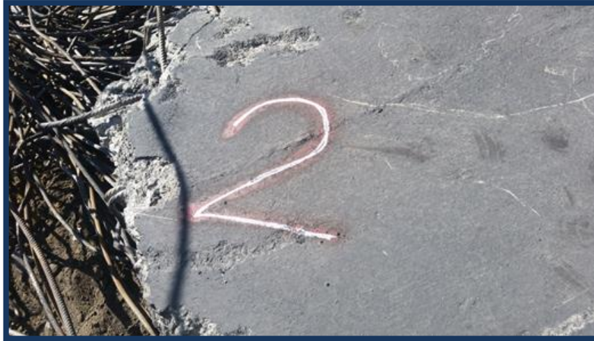
Figure 6. Part of the cylinder wall.
