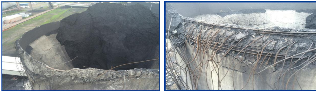
Figure 4. The part of the silo below the 25.5 m level remained in situ.
