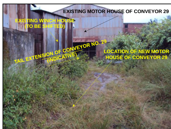
Figure 16. Tail end extension and new drive house location for conveyor 29.
