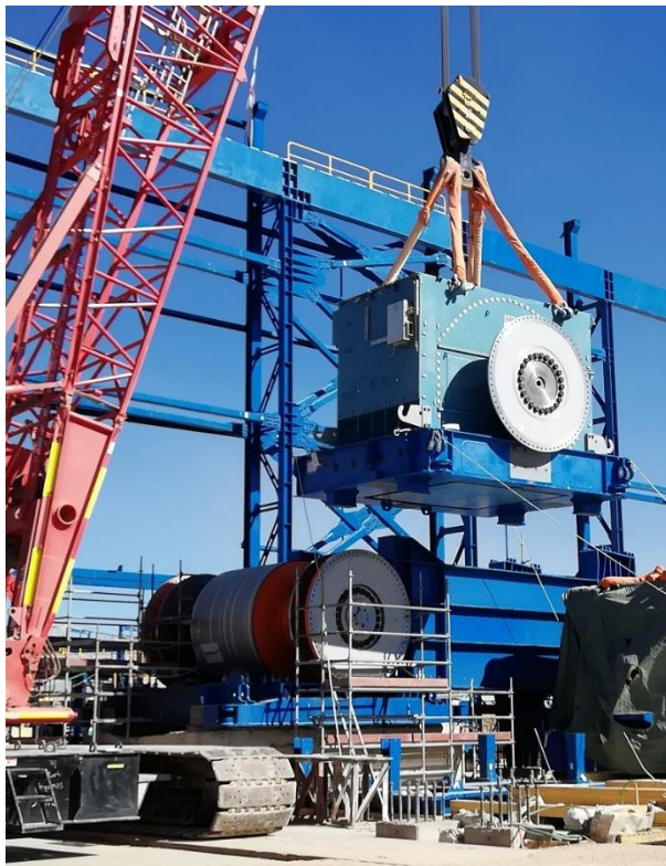
Figure 9: 900 kNm drive unit during construction
