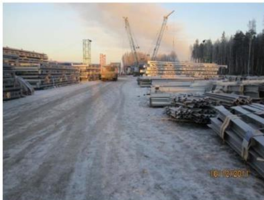
Figure 14: Assembly site of the bridge segments.
