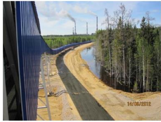
Figure 7: View of the pipe conveyor during summer.
