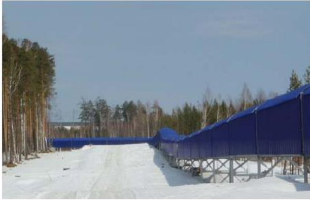
Figure 6: View of the pipe conveyor during winter.
