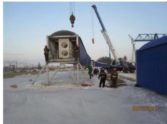
Figure 15: Lifting the pre-assembled bridges.
