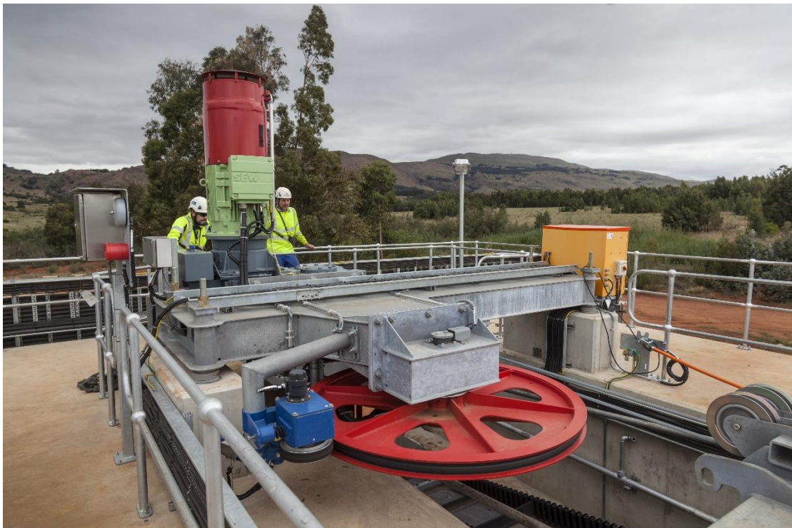
Figure 15: Inspection Carrier drive used as winch to install track rope line equipment.
