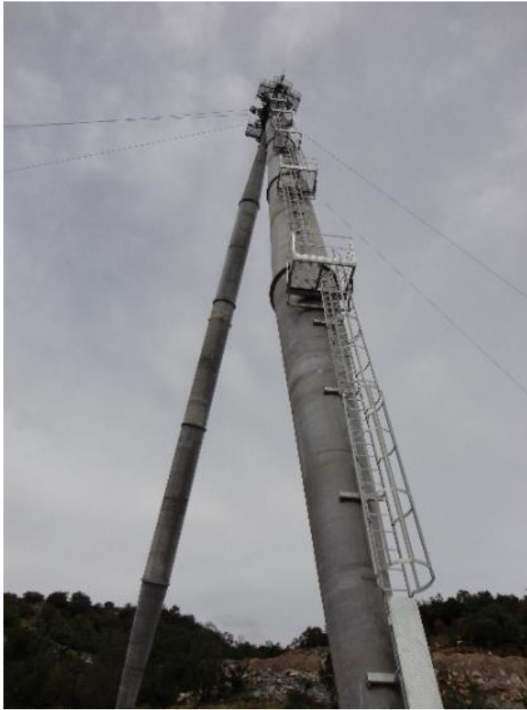
Figure 29: MHSA compliant cat ladders.
