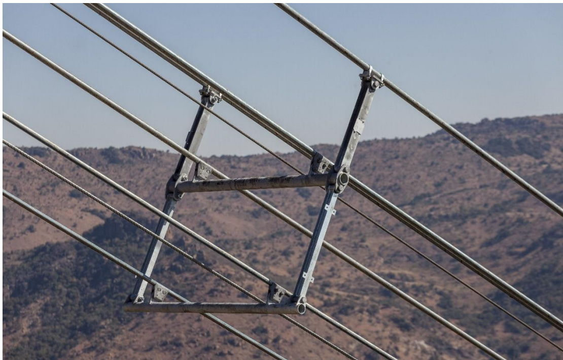
Figure 18: Installed track rope frame.
