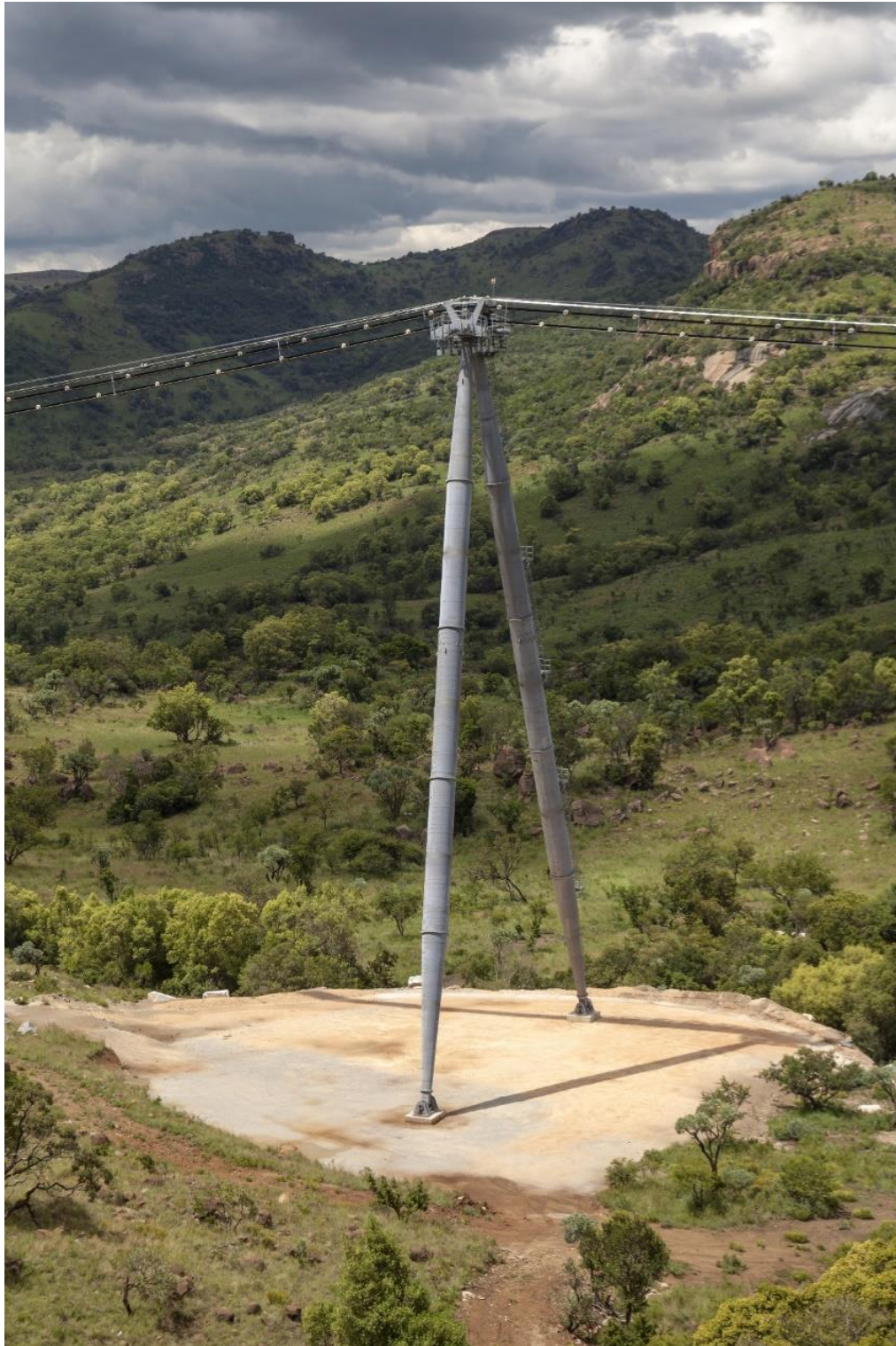
Figure 12: Tower 5, a typical A-frame tower.
