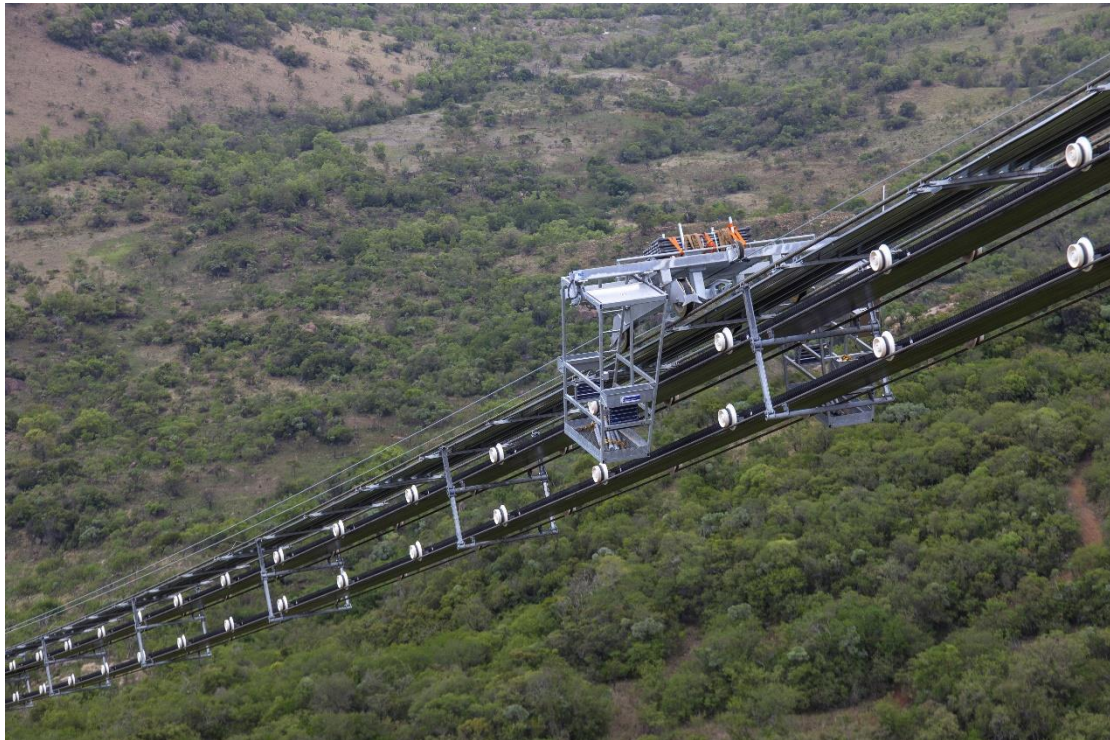
Figure 8: The BYC RopeCon Inspection Carrier with cages for personnel on both side of the RopeCon.
