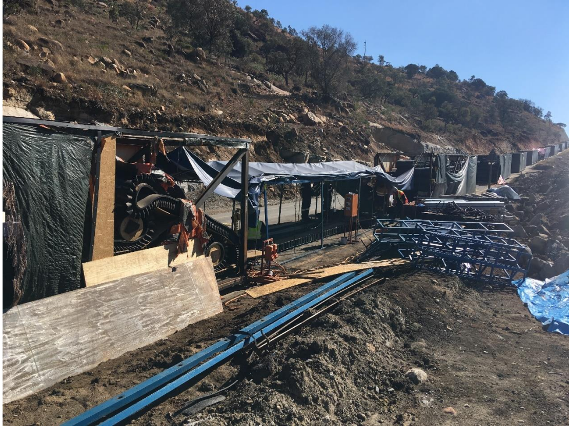
Figure 22: Splicing station set up between belt racks.
