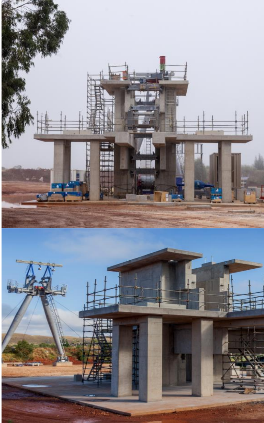
Figure 25: Intricate drive station civils cast in one continuous pour.
