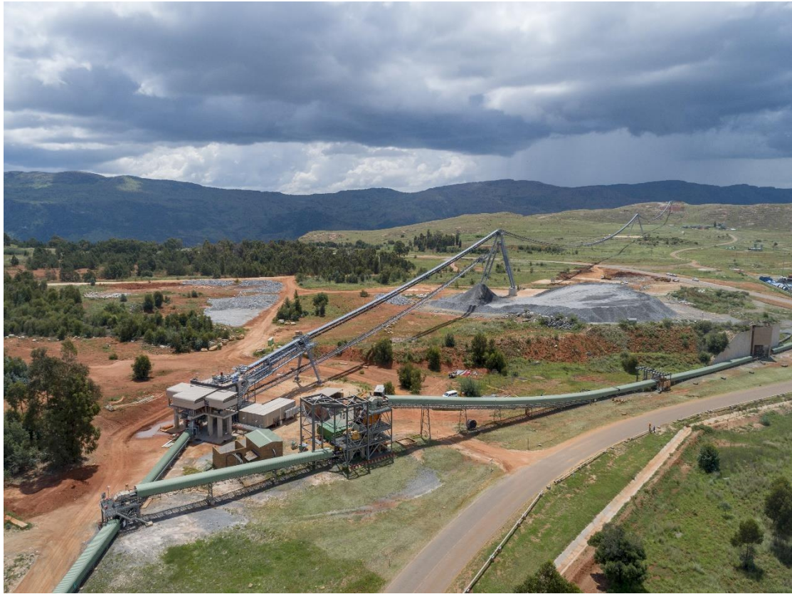
Figure 23: RopeCon unloading and drive station feeding unto the existing conveyor infrastructure.
