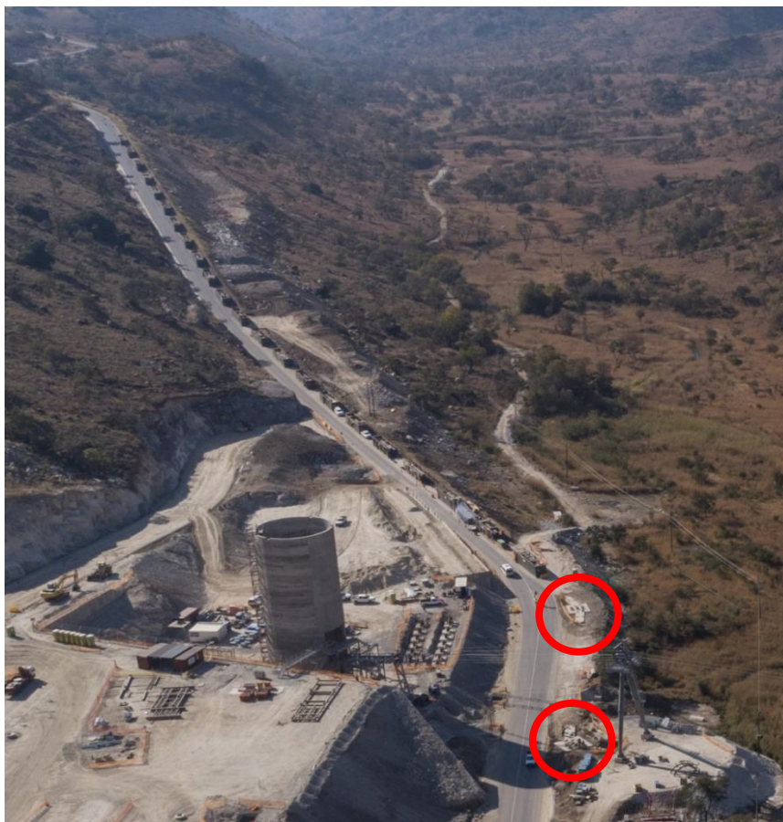
Figure 21: Belt racks placed in the road with belt deflection devices indicated in red.
