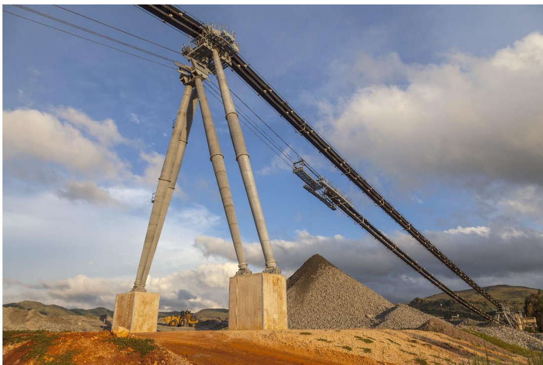
Figure 24: Tower 11 (a) and (b) with the Stock Pile Feeder head pulley suspended above the stock pile.
