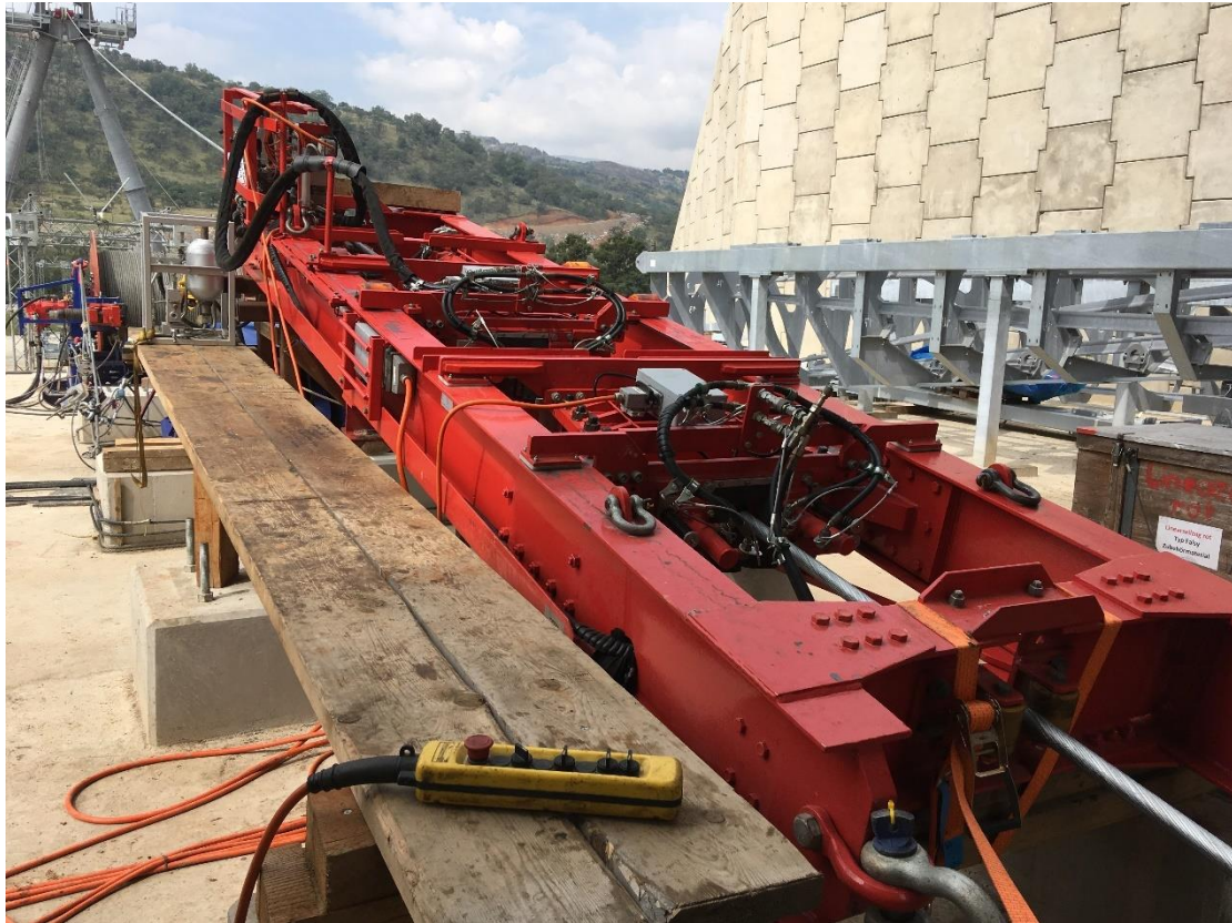
Figure 17: Specialised rope push-pull equipment used to pull the track ropes.
