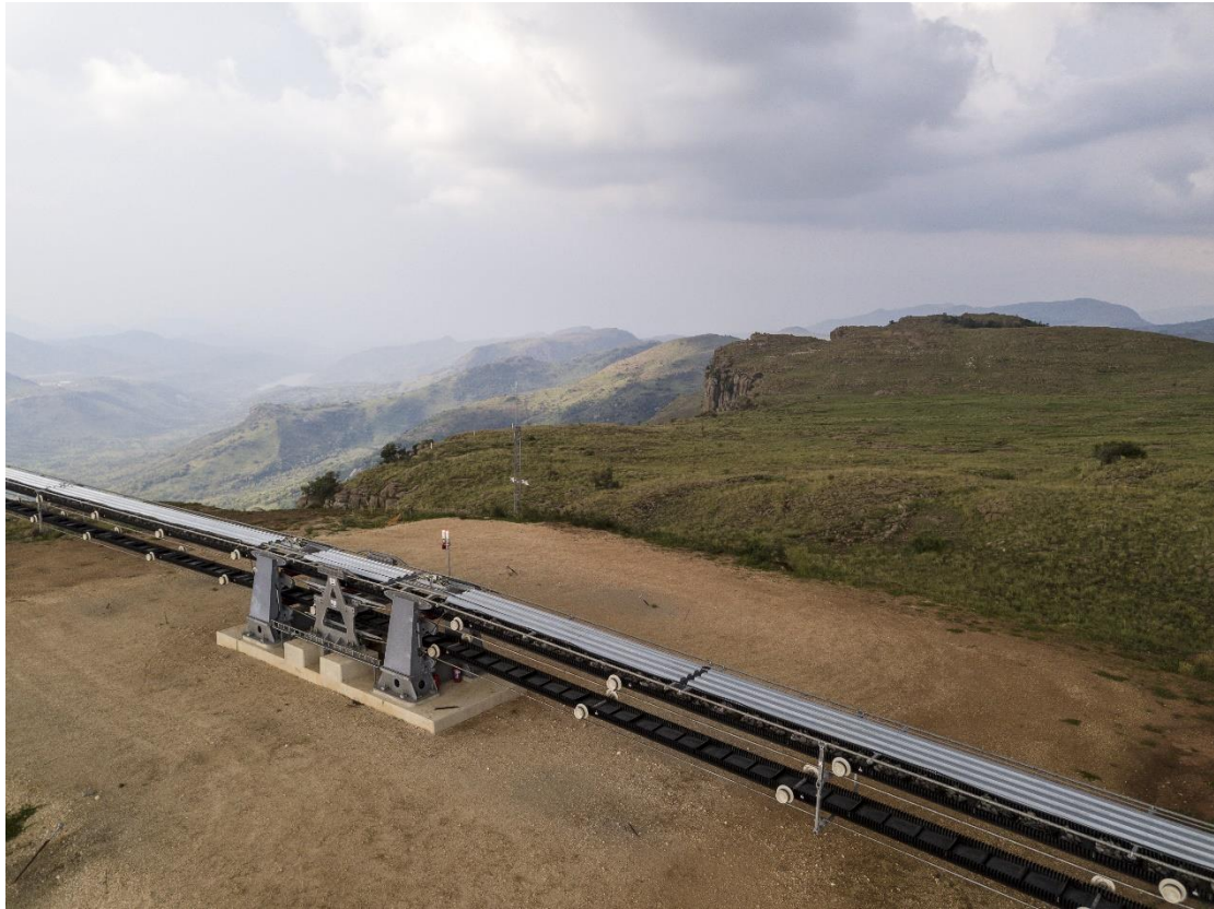
Figure 13: Tower 8, a typical track rope anchor.
