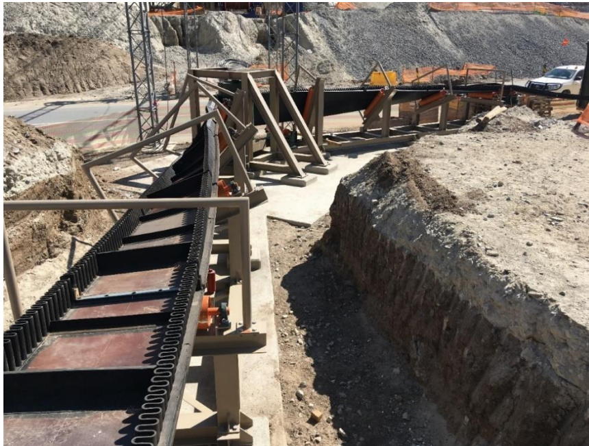
Figure 20: Belt deflection device installed.
