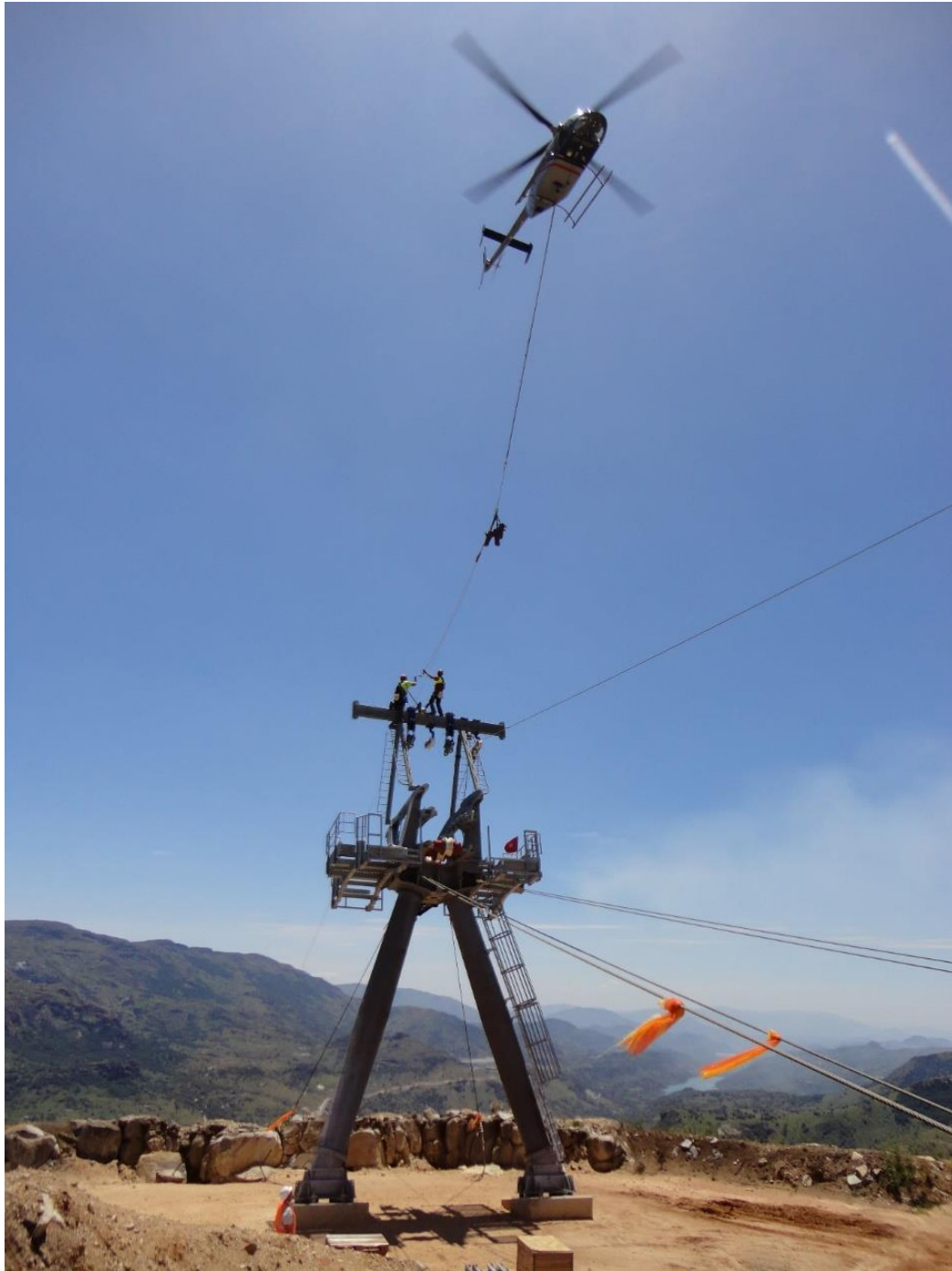
Figure 16: Helicopter pulling nylon rope up to Tower 7.
