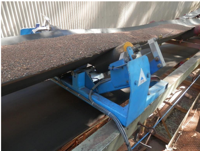
Figure 4 Conveyor belt flexure on a loaded conveyor with low belt tension.
