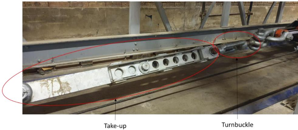
Figure 7: Take-up and Turnbuckle used to Pre-Tension the Belt
