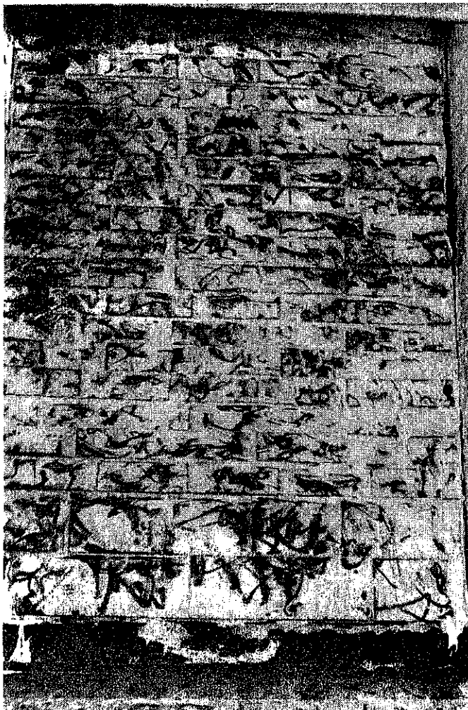
SMALLER (150 X 100 MM) TILES IN THE AREA BELOW THE FLOP GATE
