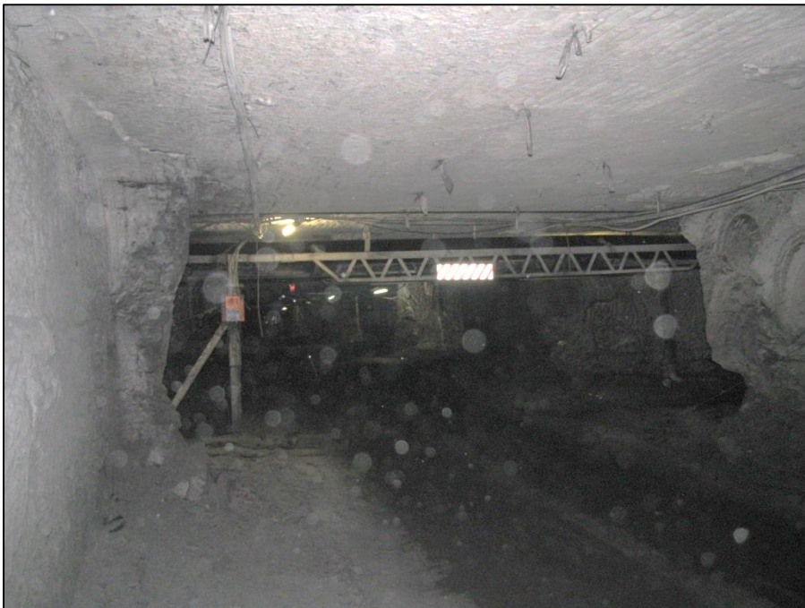
Figure 7. Image showing the bridge where the HPI took place
