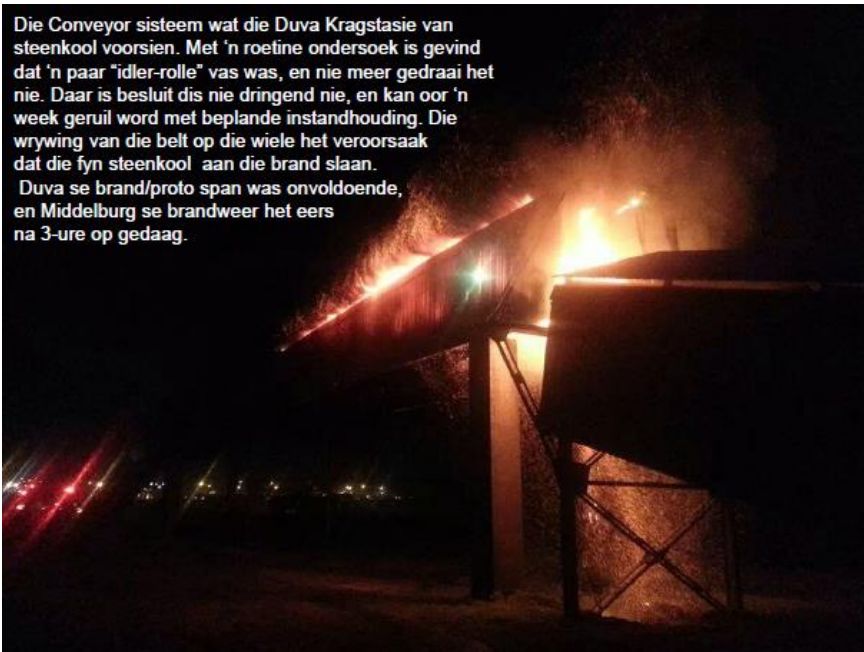
Figure 2. Conveyor fire at Duva Power Station
