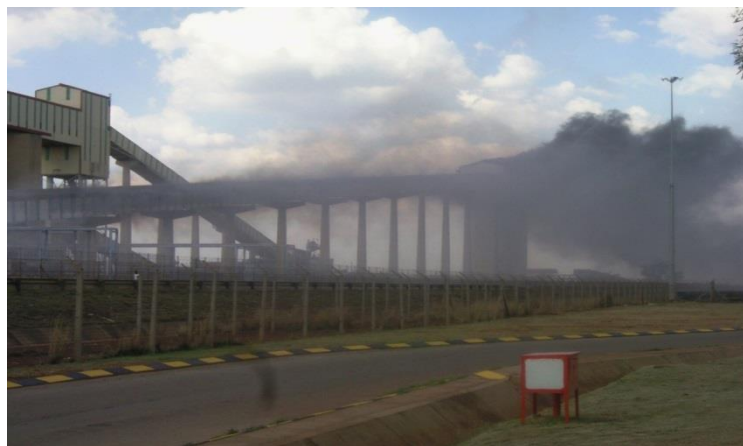
Figure 1. Conveyor belt fire
