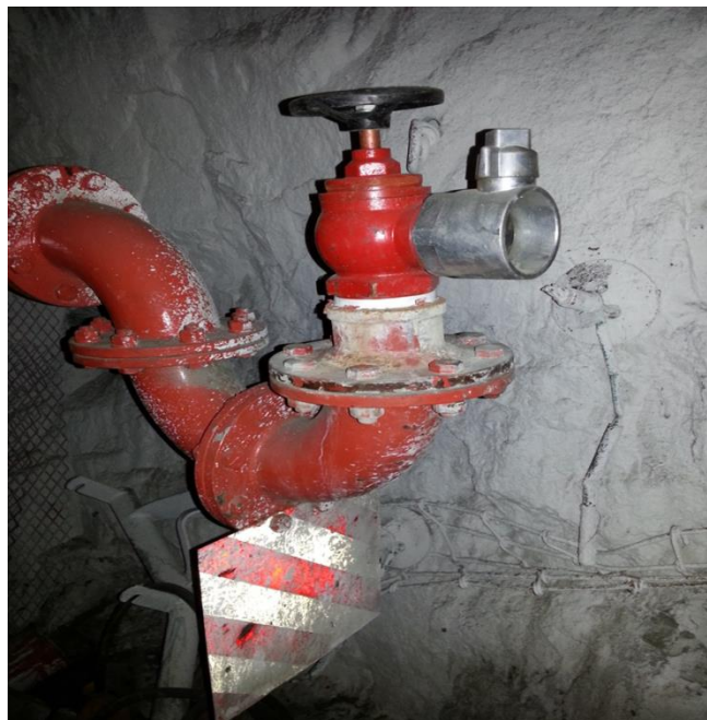
Figure 13. Fire hydrant
